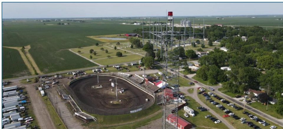
The guy that put the telephone tower up forgot to put any transmitters or antennas on it. He'll get a great view of the races when he comes back though.
